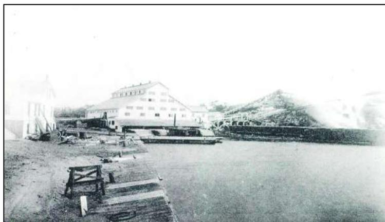
Figure 6. The new four-storey mill was constructed in 1878 to 1879 at the man-made opening of the Musquash River on the eastern side of the Mill Island. Conveyors, which can be seen in this image, carried sawdust from the mill to the two sawdust bays on either side of the mill.
