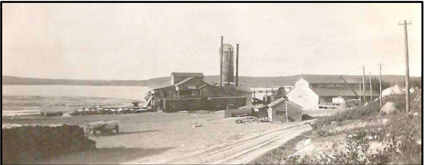
Indian Lake Lumber Sawmill at Osaquan - Planer Mill is to the right
