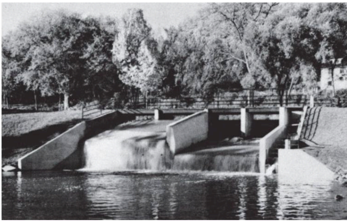
The Owen Sound Mill Dam on the Pottawatomi River was restored in 1959 by the North Grey Conservation Authority; to the right of the dam can be seen the first fish ladder constructed in Ontario.
